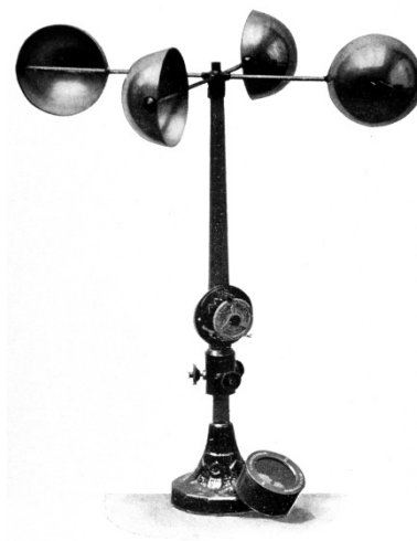
THE ROBINSON ANEMOMETER.
